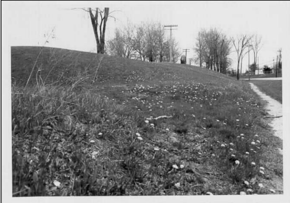
Figure 3: Fort Brown, Plattsburgh, Clinton County, New York View: NE along parapet.
