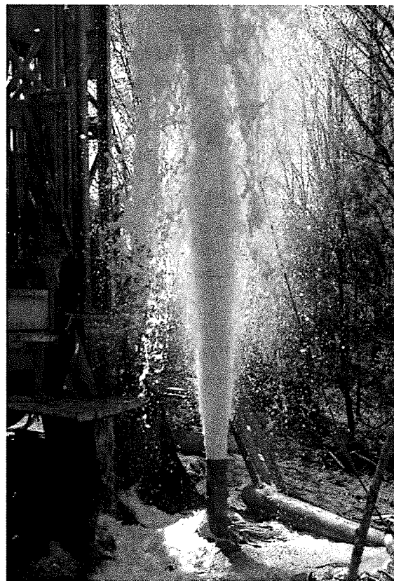
Installation of an HSA-sited test well
