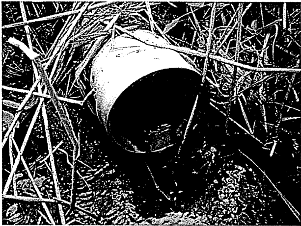
Stone identified the presence of dry weather flow at a wastewater pump station, suggesting that a municipal water leak was infiltrating the pipe (contributing chlorine) and flushing out wastewater residues from past overflow events.
