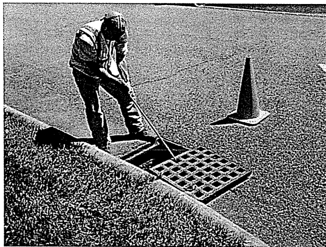
Stone scientist inspecting a catchbasin for dry weather flows.
