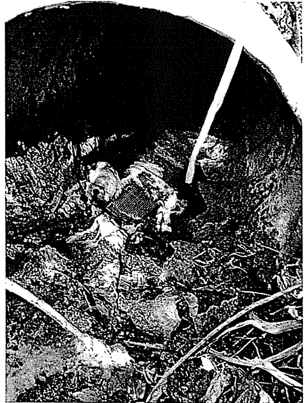
Toilet paper caught on a monitoring pad in a Rutland Town outfall. Hotel management eliminated the cross-connection in 2018.
